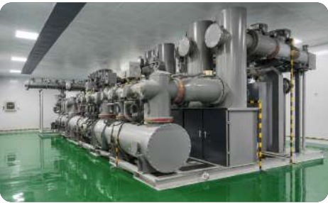
Prefabricated HV GIS
