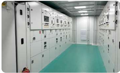
Prefabricated Switchgear
