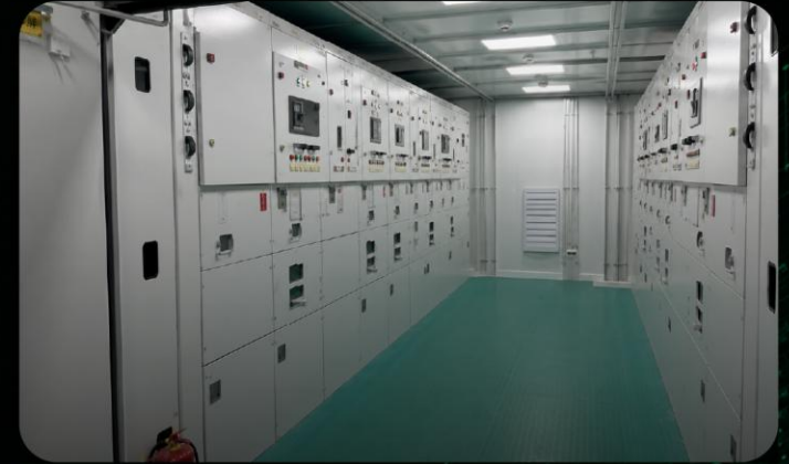
Prefabricated Switchgear
