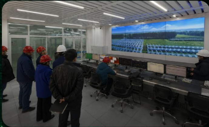
Prefabricated Secondary Equipment
