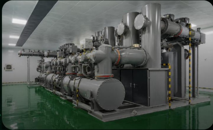
Prefabricated HV GIS
