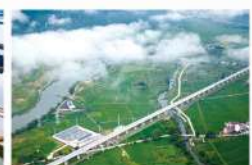
Changjing-Huangshan High-Speed Railway
