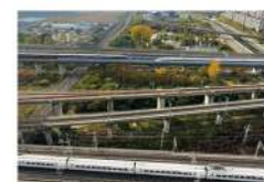
Beijing-Shanghai High-Speed Railway
