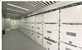
0.4kV - 35kV Prefabricated Switchgear Cabin
