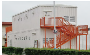
0.4kV - 35kV Prefabricated Switchgear Cabin
