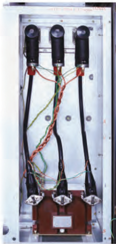
Potential Transformer Connection Section
